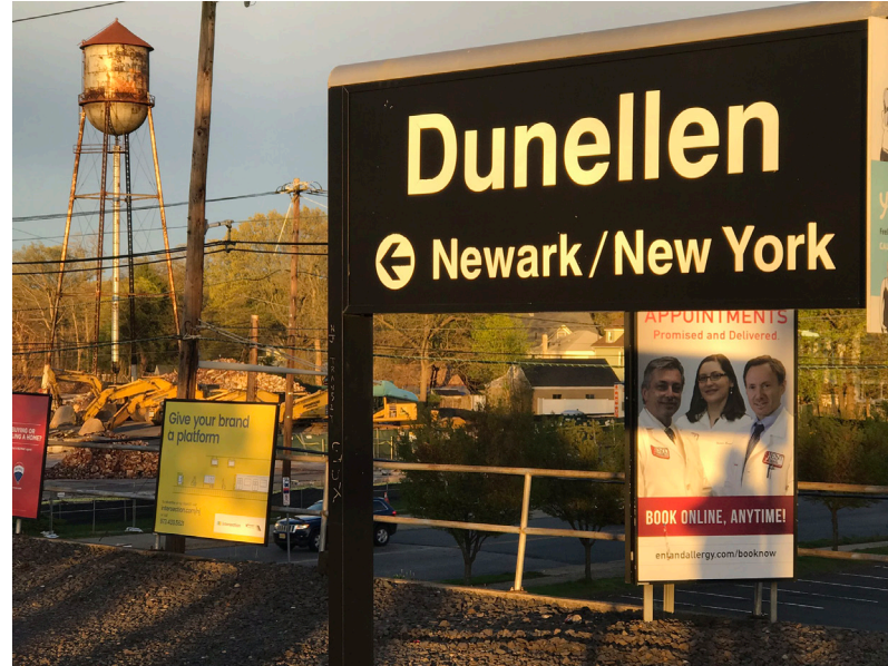
Top: The historic Art Color Printing Co. water tower and the rubble from its demolished buildings are visible from the train platform (Spring 2019); the developer is prepping to build new transit oriented development, as shown below.
