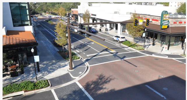
Image is an example of the Complete Street concept utilized on Swann Avenue n Tampa. Source: www.tampagov.net .
