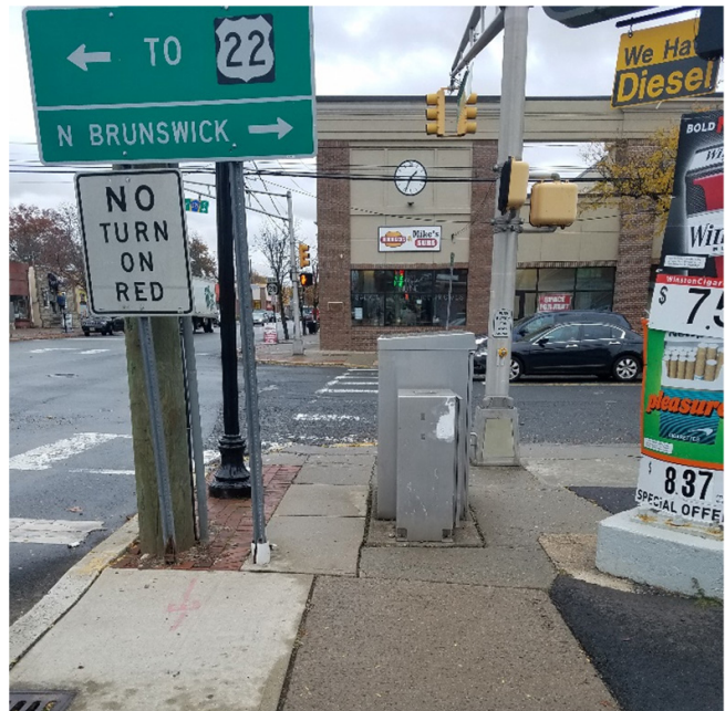
At the southwest corner of North Ave and Washington Ave, the large metal cabinet signal control box reduces the width of the sidewalk.
